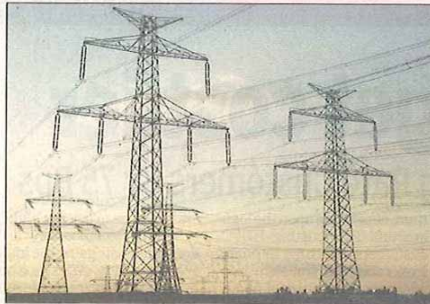
DECKS CLEARED FOR EXPANSION
